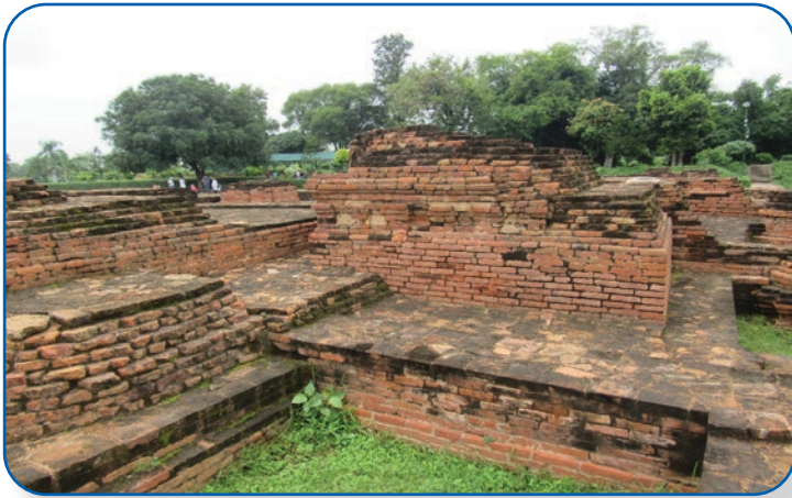
A ruined foundation
