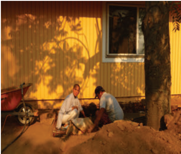
Chánh Đức Minh made a toilet tunnel for Hương Sen Temple
