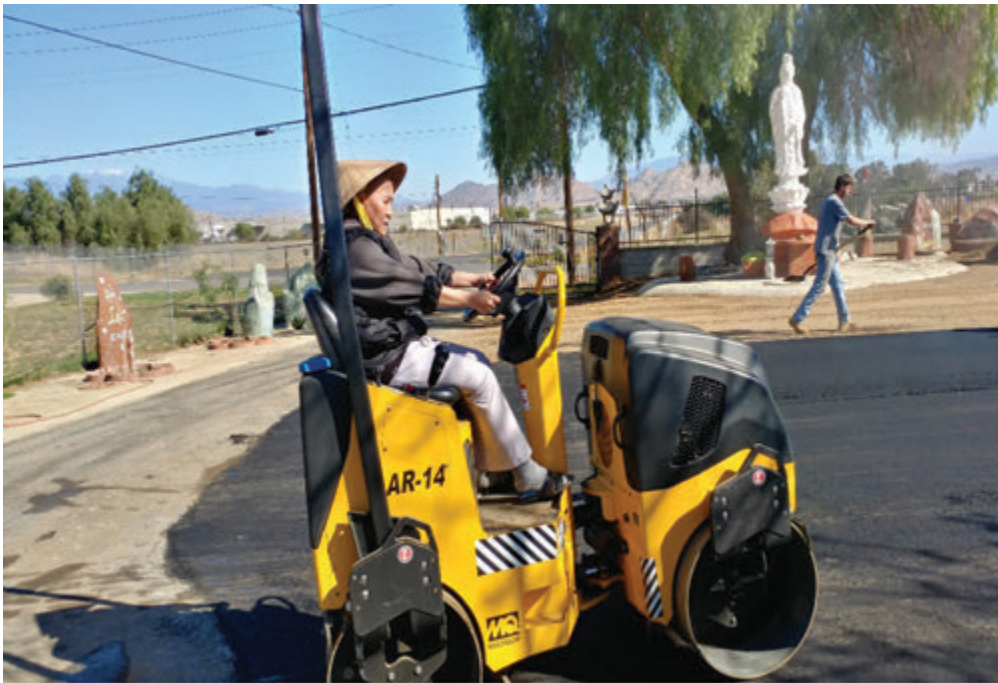
Making the parking lot, 2016
