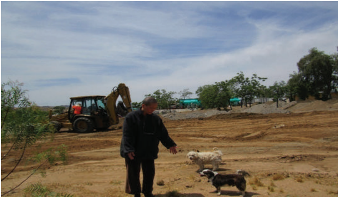
Leveling the soil to build the temple ground, 2013
